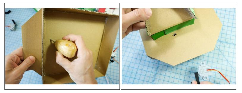
Make holes in the box to thread the motor wires through. Place the fish body on the plaque to find the correct location of the holes.
